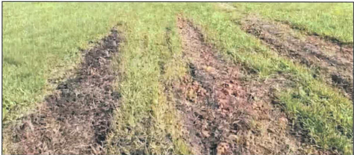
Figure 5: Efogi airstrip damp wheel bogging track
