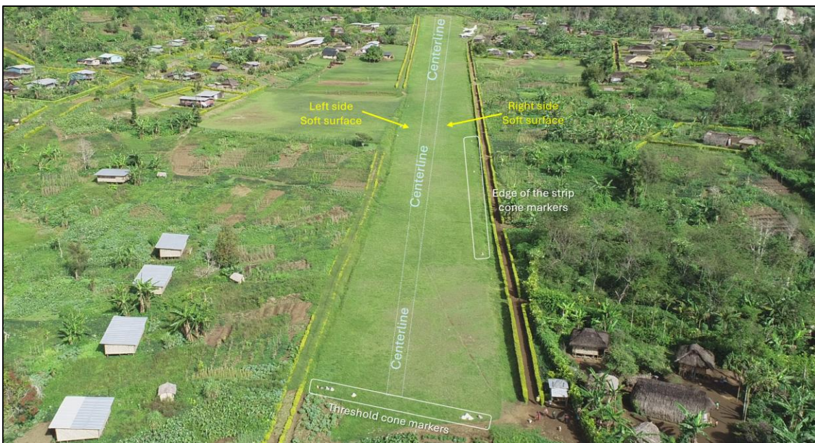
Figure 8: Bungawat Airstrip with indications of the on-site team observation
